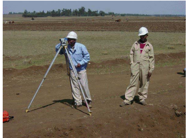
Fig.4: Ethiopian colleagues levelling for a (Japanese financed) road project in the Ethiopian highlands
