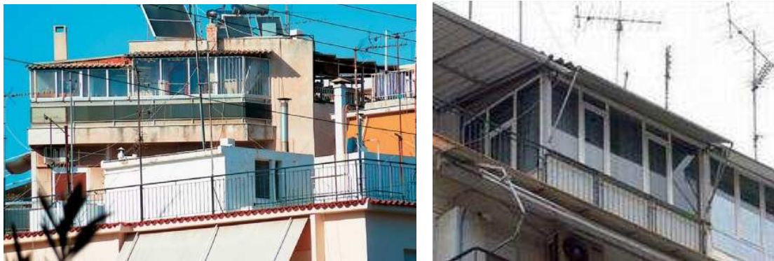
Figure 2. Informalities in the planned areas that do not exist within the ratified outline of the volume of the building, but can be formalized by Law 4014/2011
