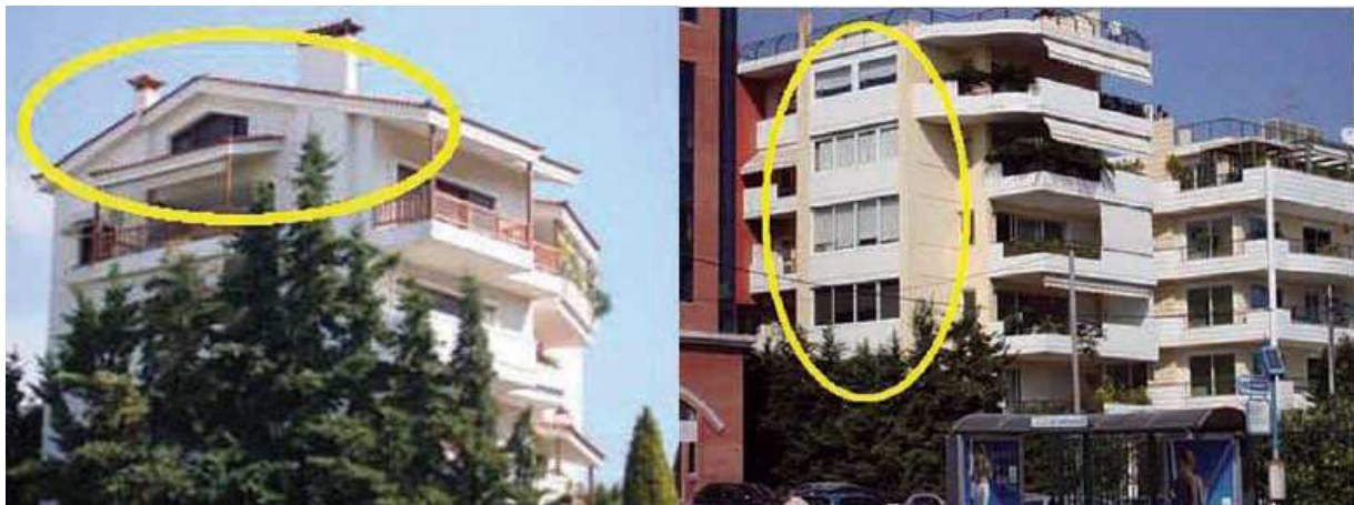
Figure 1. Illegal room under the roof of the building (left); build-up semi-open areas within the ratified outline of the volume of the building (right). Source: (Dimopoulou et al, 2007)
