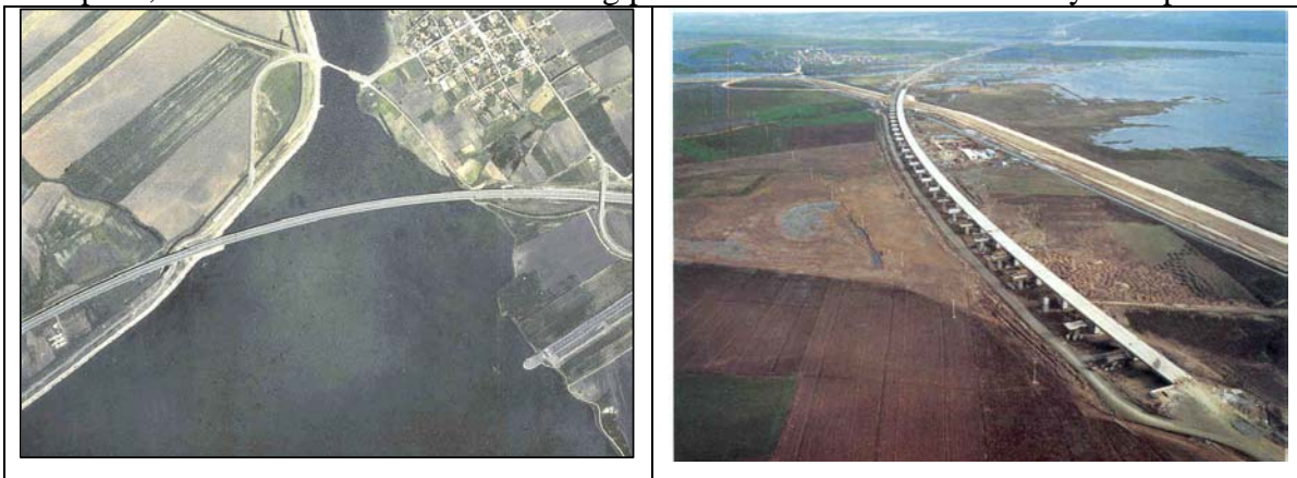
Figure 1: The Karasu viaduct
