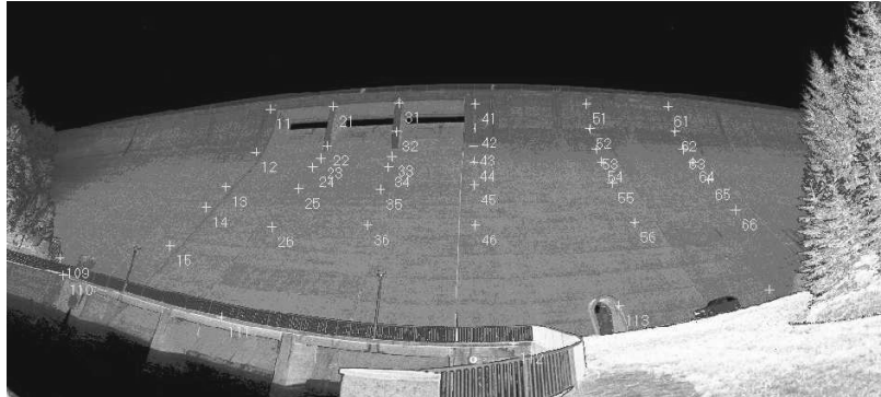
Figure 12: Intensity image of dam Rauschenbach incl. check points
