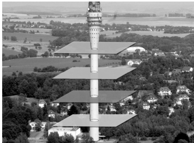
Figure 6: Cut of the point cloud into thin layers and projection onto 2D planes
