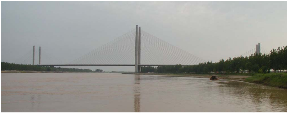
Figure 1: Shandong Binzhou Yellow River Highway Bridge
