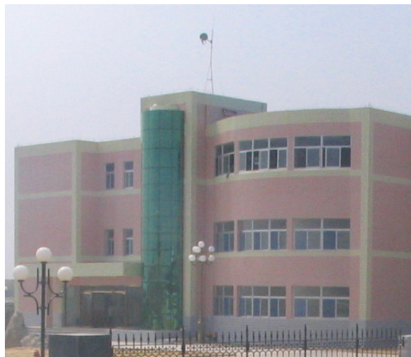
Figure 12 Wireless Bridge installed in RBMC
