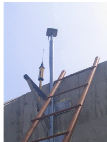
Figure 7: GPS sensor mounted at the top
