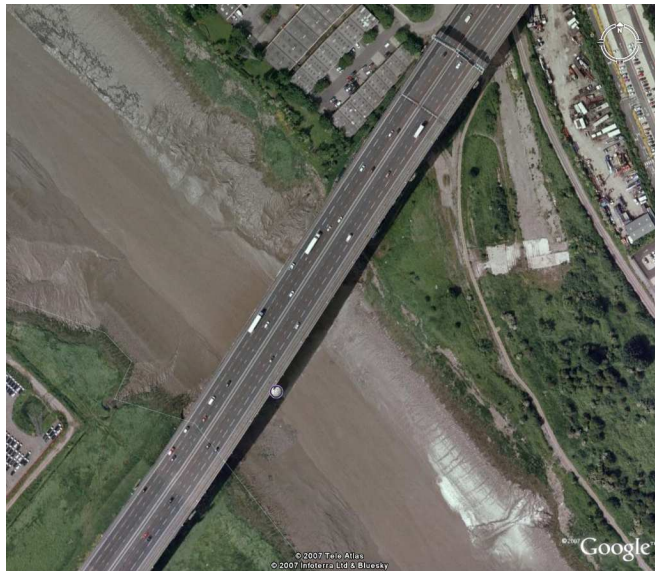
Figure 2 - A Google Earth image of the viaduct.
