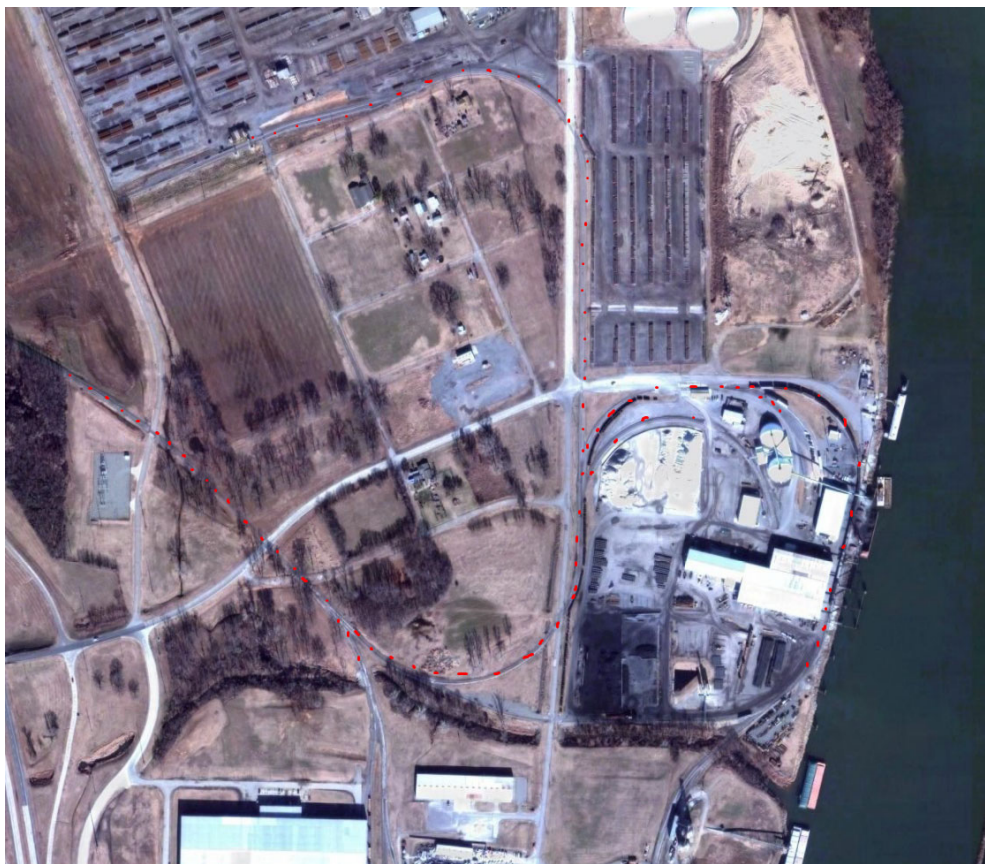
Figure 1: Rail corridor surveyed by Lynx Mobile Mapper outside Tulsa, Oklahoma
