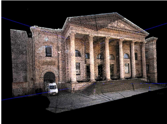
Figure 14: Results of a terrestrial scanning of a complex facade
