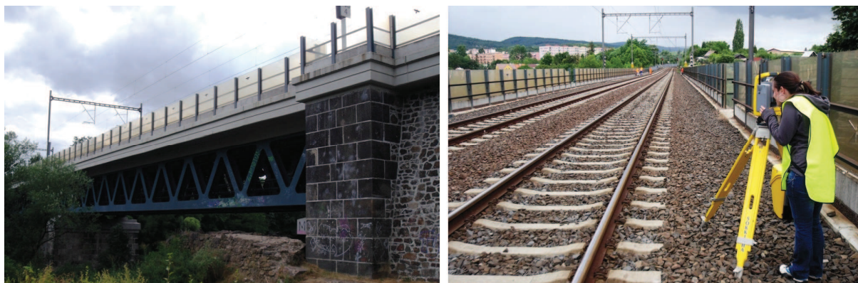
Figure 3 Railway bridge in Klášterec nad Ohří
