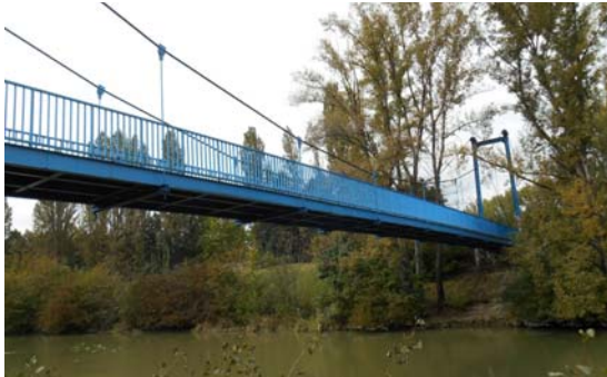
Fig. 3 Pedestrian bridge over the river Malý Dunaj in Bratislava, Slovakia
