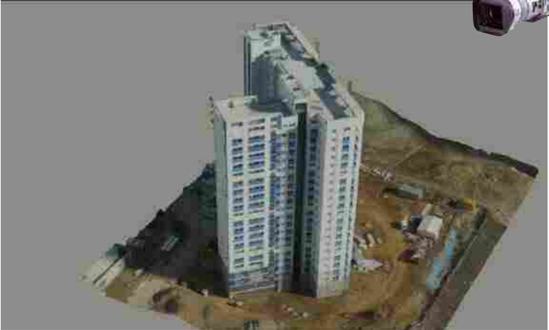
3D modeling / Safety inspection
