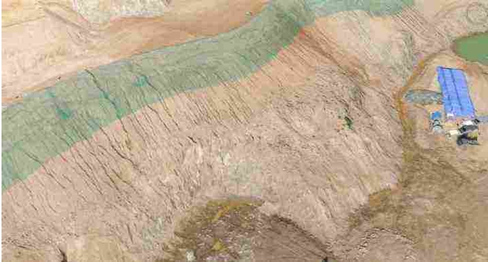
Slope safety management
