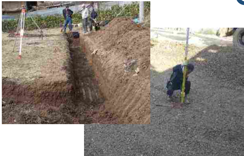
Excavation location, depth verification etc.
