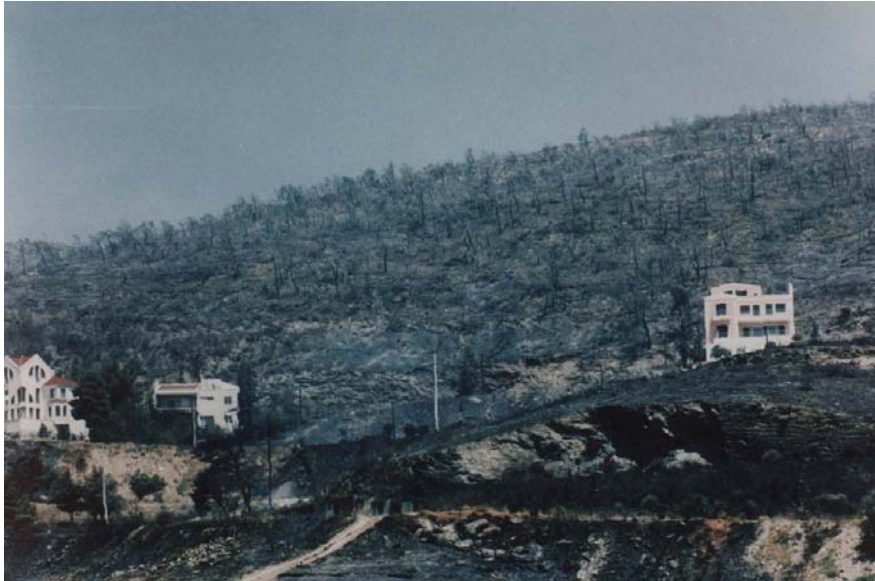
Figure 5. Informal buildings within forest land; situation after a big fire in eastern Attika
