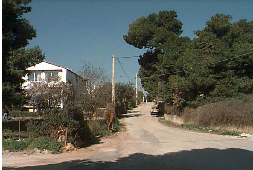
Figure 2. Area under legalization process (Rafina, Attika); electricity connection is provided
