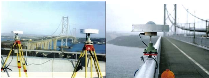
Fig. 2. Two GPS reference receivers located adjacent to the Forth road bridge (left). A GPS choke ring antenna attached to the bridge (right).
