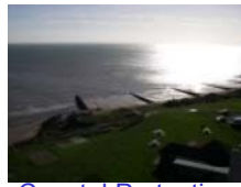
Coastal Protection & Development
