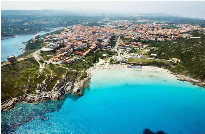
Fig.3 - Results of unfettered building development
