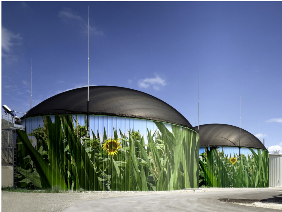
Figure 4: Concept study for a biogas plant (Source: Fachagentur Nachwachsende Rohstoffe e.V. (FNR)).
