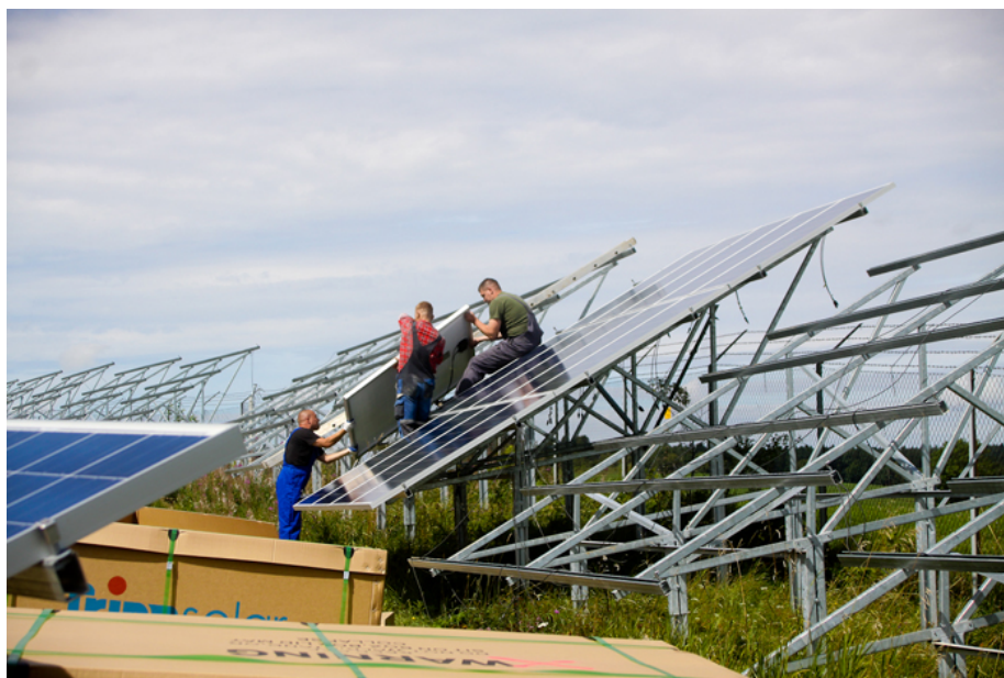
Figure 10: Construction of a solar energy plant (Source: die STEG Stadtentwicklung GmbH).
