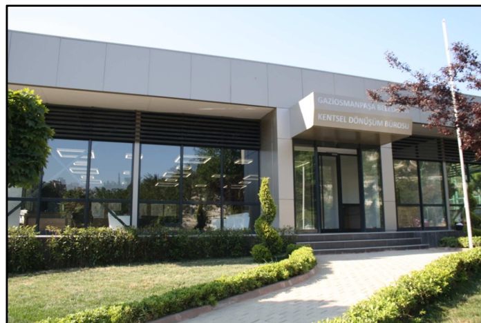
Figure 11: Sarıgöl Neighborhood Urban Regeneration Office
