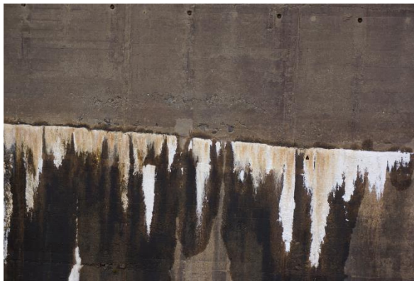
Figure 24 – Horizontal photograph of the downstream wall of Bouça dam.
