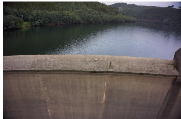
Figure 25 – Inclined photograph of the spillway on the crest of Bouça dam.
