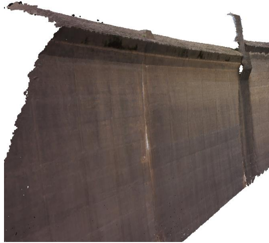
Figure 26 – Point cloud of a section of the spillway.
