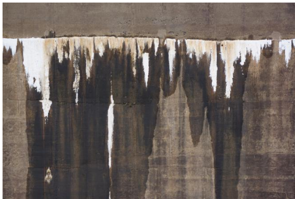
Figure 27 – Flight A. Central crack photographed with a focal length of 50 mm.
