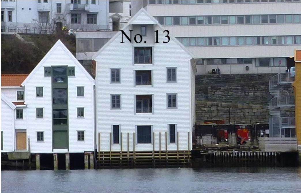
Figure 11. Skuteviksboder no. 13 after reconstruction in 2014. No. Photo: Leiv Bjarte Mjøs
