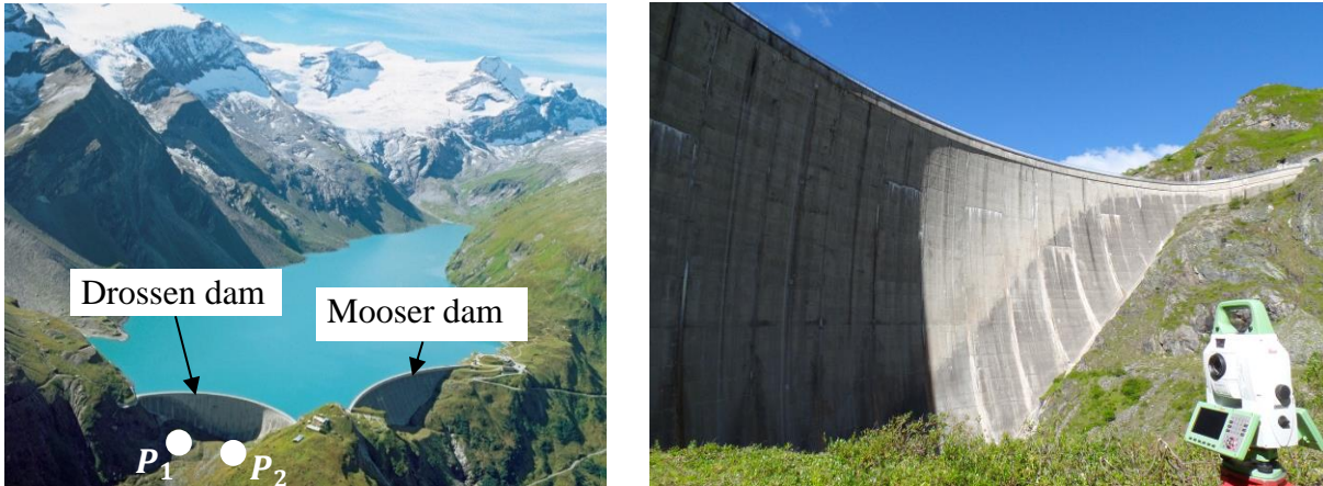
Figure 2: Measurement site, overview image showing the two concrete dams of the reservoir Mooserboden (left, source: Verbund), frontal view on the downstream side of the Drossen dam with the instrument set up at point P_1 (right)
