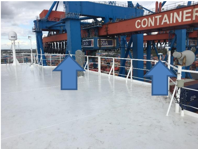
Figure 4 Wheelhouse Top over the navigation bridge
