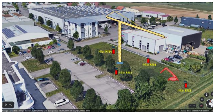
Figure 5: Isometric view of the real-world construction area (based on data from Google Earth 2022)
