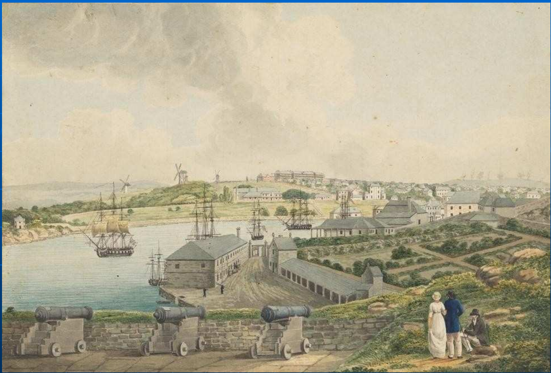
VIEW FROM DAWES POINT BATTERY TOWARDS THE EAST
